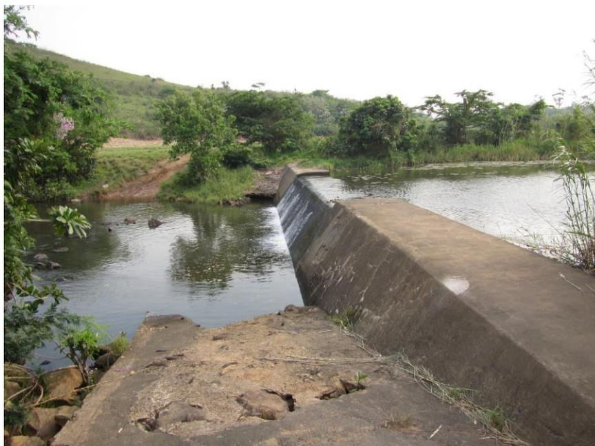
**Figure 1: The weir on the Ntuze tributary. The water dammed up by the weir is used as a back-up supply for the town of Mtunzini. In the past the tidal ebb and flow point was upstream of this point. Nowadays this is the upper reach of the estuary on this tributary.**
